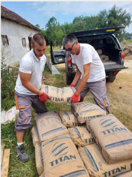
EULiBOR technicians helping build a water-access project in Lukavac Village.
