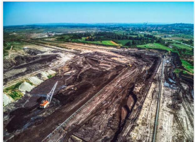
Existing open pit coal mining operation in the Kolubara District.
