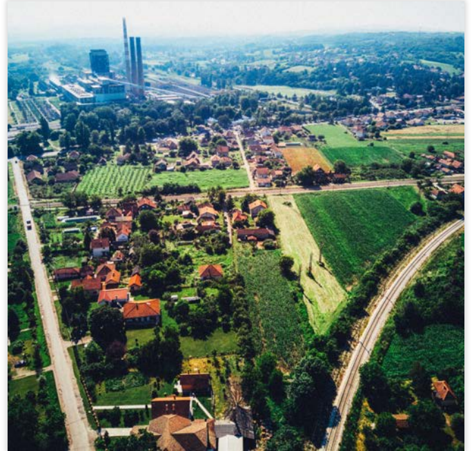
Local coal-based thermal power plant.
